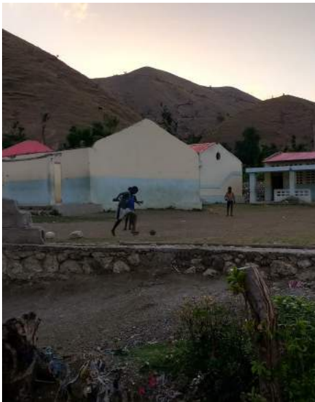
Roofless public school, Côteaux, February 2017
