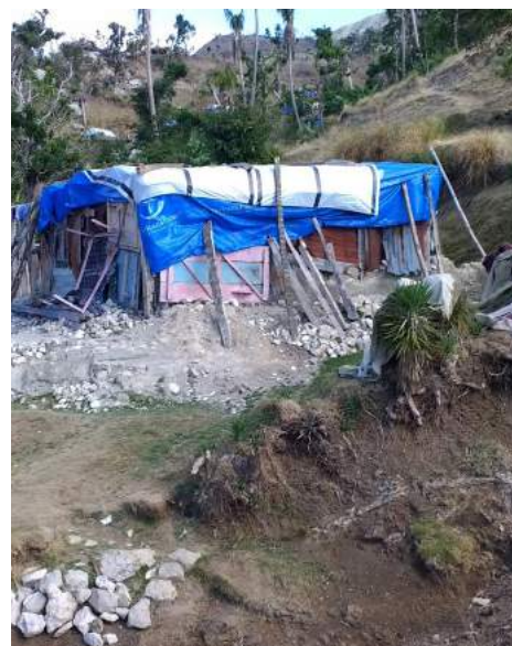
Destroyed home in Côteaux, February 2017
