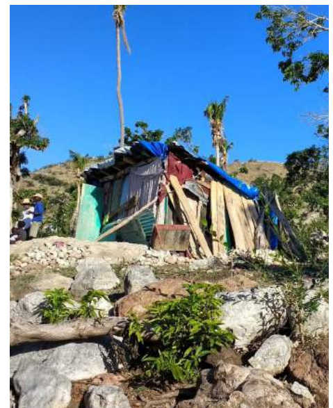
Destroyed home in Digo, Côteaux, February 2017
