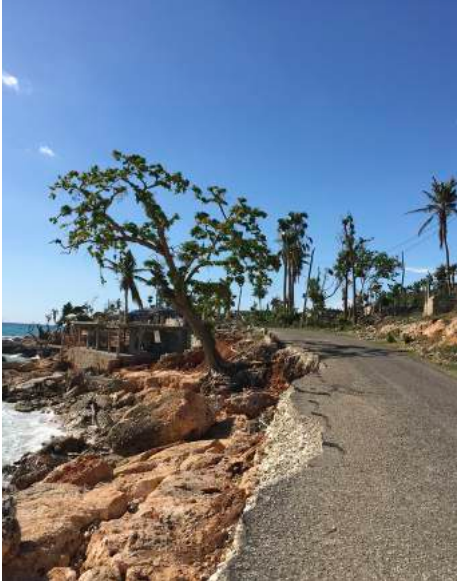
Damaged road in Port Salut, February 2017
